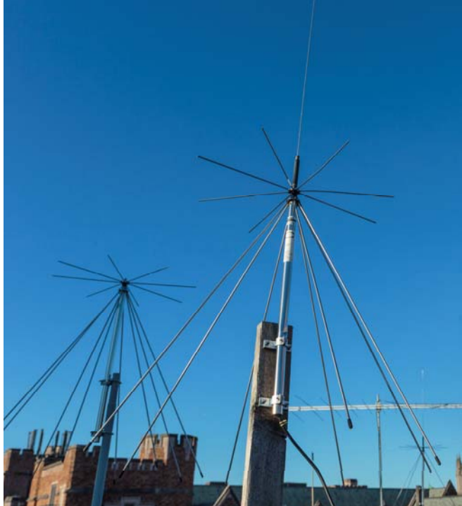
Installation on the rooftop of Sieg Hall, UW
