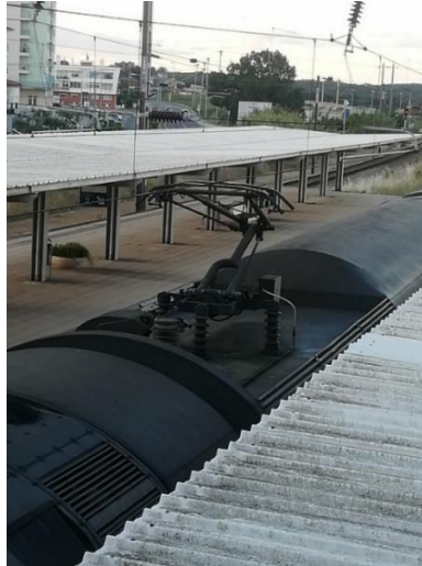
Figure 3.12 Pantograph and Catenary – Azambuja's station.
