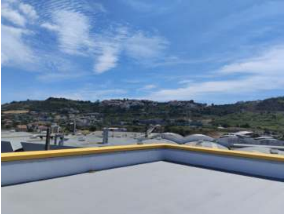
Figure D.2: NOS BS view of the rooftop in front of the measured sector.
