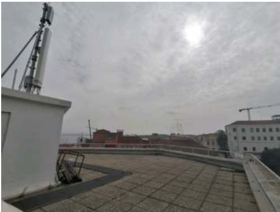
Figure D.4: MEO BS view of the rooftop in front of the measured sector.
