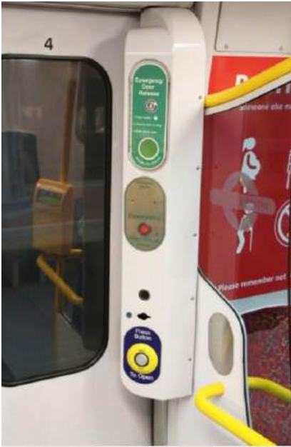
ECS Emergency Call System
